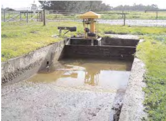
Photo 16: Trafficable sump with Rankin pump at the Vasse Research Station (courtesy Rob Summers, Department of Agriculture and Food).
