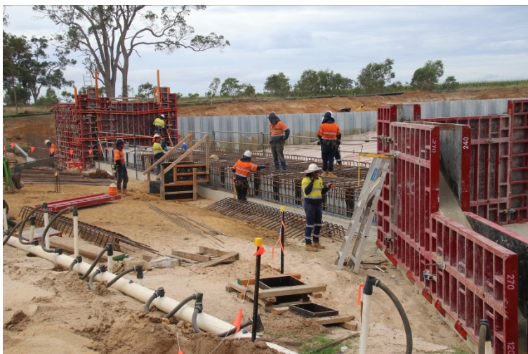
Construction of the culverts
