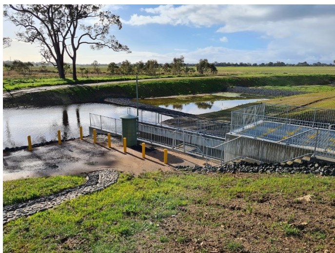
The diversion drain and upgraded culverts
