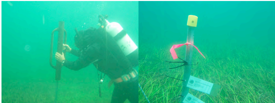
Figure 2: Left: Banging in permanent marker with pole driver. Right: Star picket with cap and plastic coated site label, indicating centre of 50 m diameter Keep Watch seagrass site.
